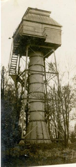
**The Azimuth Instruments were used to determine the “bearing” (angle) to any enemy ship in the bay or in the Patapsco River shipping channel. The soldiers in this tower and those in a second Base End Station across the river at Fort Smallwood would take bearing measurements simultaneously. See the picture below.**
