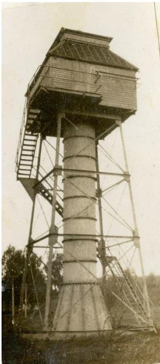
**This tower was the communication hub for the entire harbor defense when the big guns were in action. Overall control of the guns and underwater mines would have come from here. The officers and soldiers in this tower were linked by telephone to all fire control stations and gun batteries at all four forts on the Patapsco River.**
